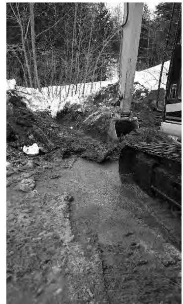
Construction of a drainage swale on Bangor Street to alleviate flooding issues
