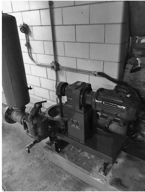
Night Soil Pump at Wastewater Treatment Plant
