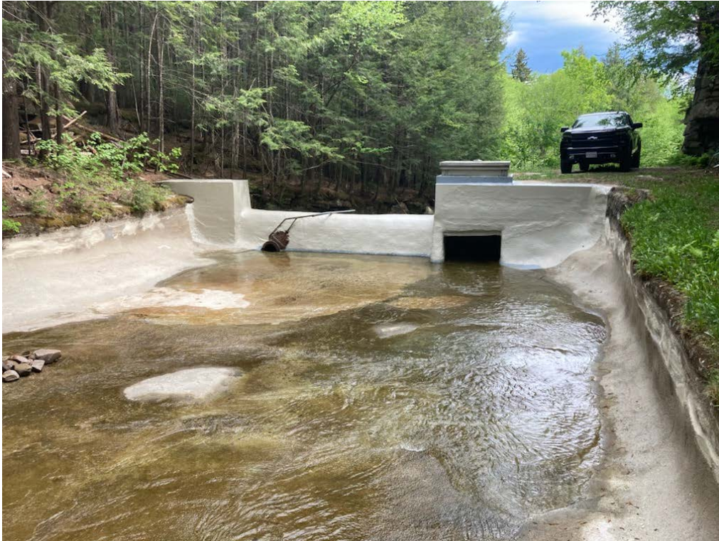
Applied Epoxy Coating to Perkins Brook Dam
