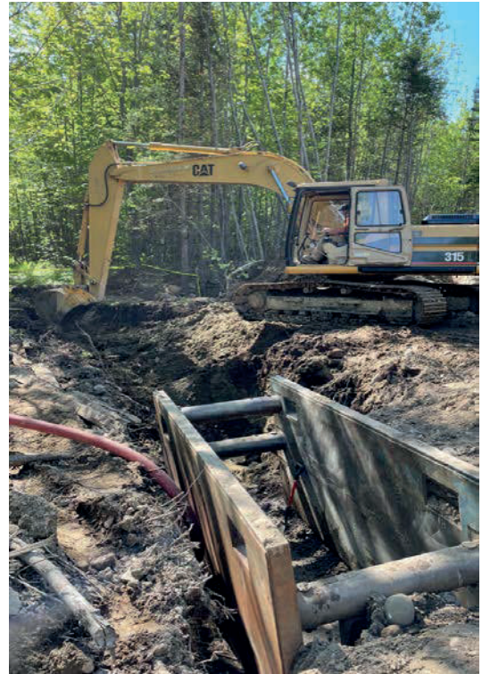
Replacement of 4" Cast Iron Water Main on Gorham Hill
