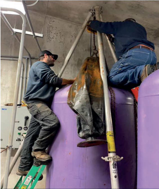
Replacement of Bladders in the Hydro Pneumatic Tanks at the Water Treatment Plant
